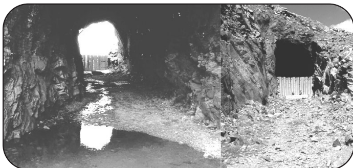
LEFT: INTERIOR OF NEEDLES EYE TUNNEL ON JUNE 26'
