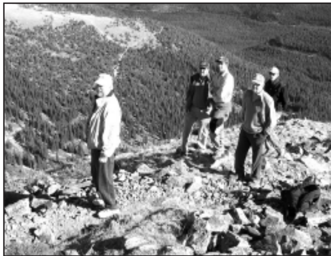
Boulder County Commissioners inspect the Devils Slide Trestles and the top of the Needle's Eye Tunnel.
